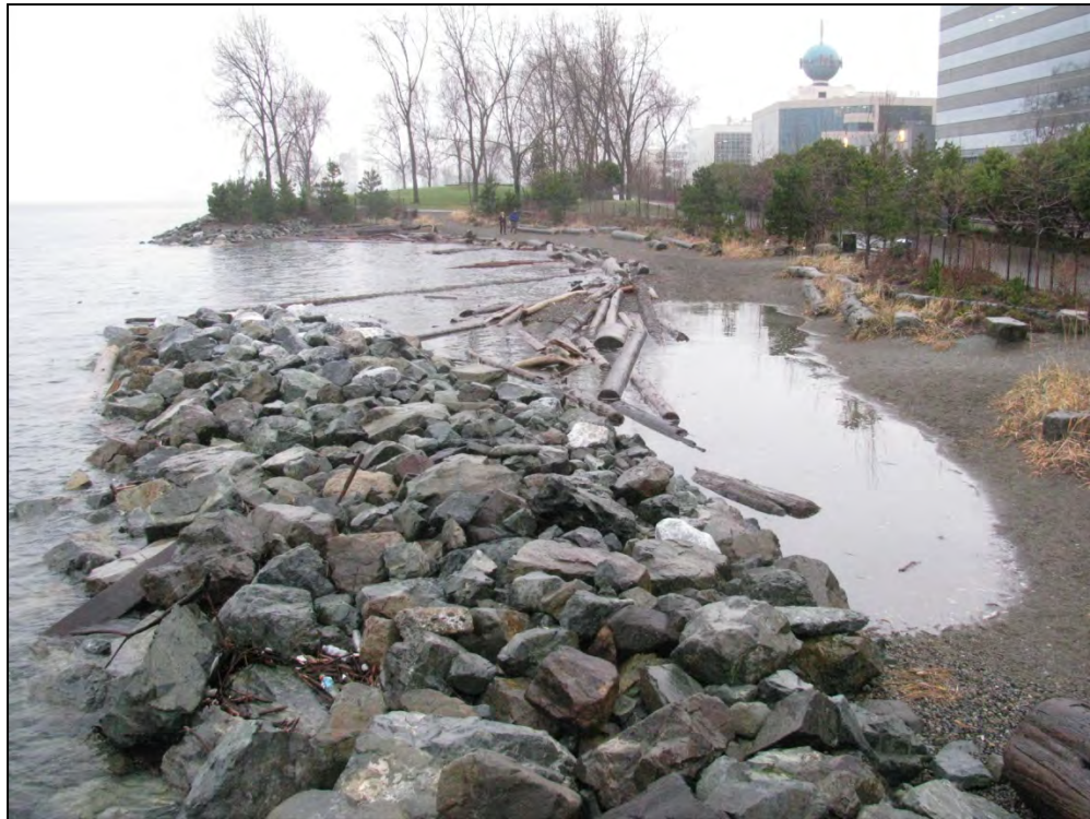
Figure A -2: A high tide event at a restored beach in the City of Seattle. Restoration projects such as this pocket beach should be selected and designed in ways that accommodate rising sea levels. Photo by Hugh Shipman.
